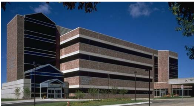
main lobby entrance
