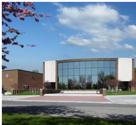
outdoor plaza renovation
